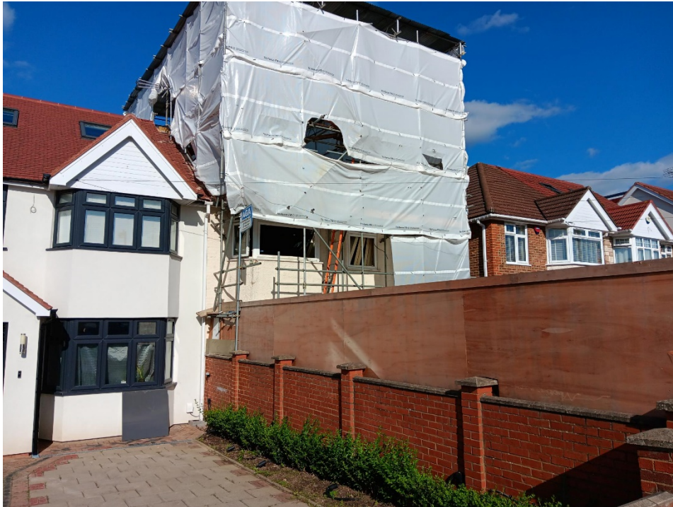
Figure 3 Front of property and adjoining semi-detached unit
